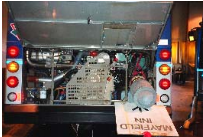
Figure 4. LFE plumbed to Engine Air Intake
